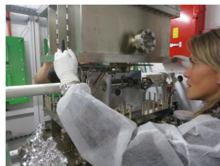
Figure 4: Installation of mirrors M1 and M2 in Optics Hutch 3.
