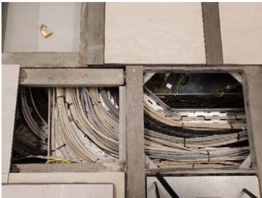
Figure 2-150: Storage Ring CIA showing underfloor cable containment.
