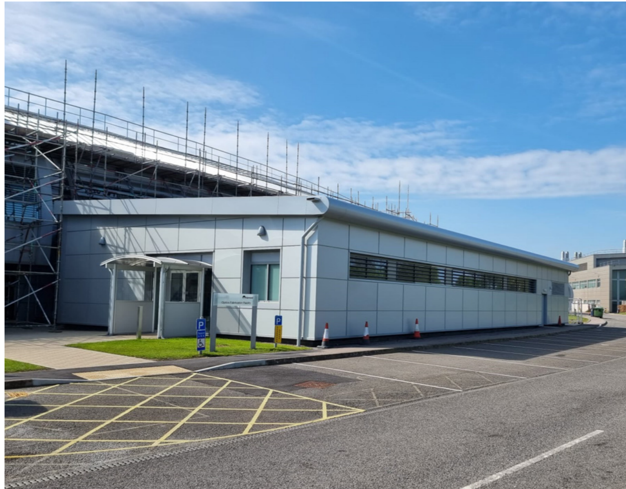
Figure 1: Optics Fabrication Building.
